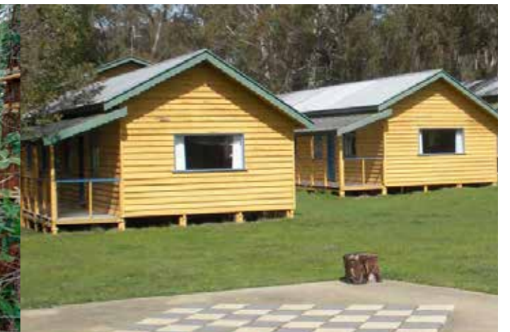
Refurbished Cabins for Camp Groups
