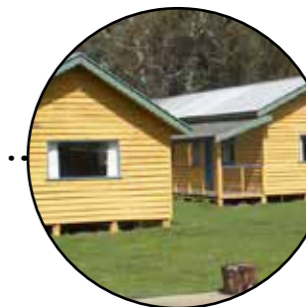
Refurbished Existing Camp Area. To be privately operated.
