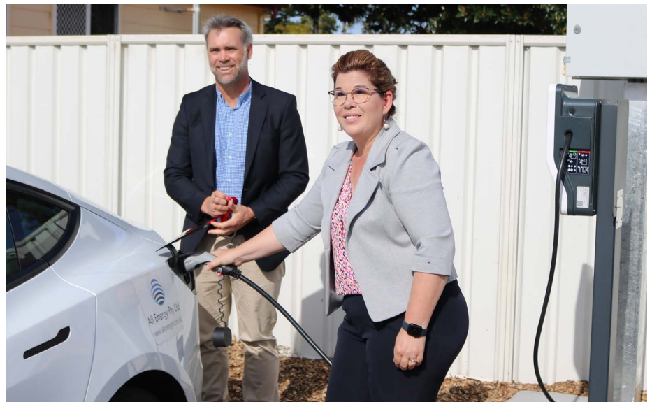
Above: All Energy Pty Ltd Lead Engineer Gareth Forde and Balonne Shire Mayor Samantha O'Toole put the new EV charger to the test.
