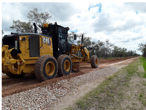
Disaster Recovery works in action on Hoolavale Rd.
