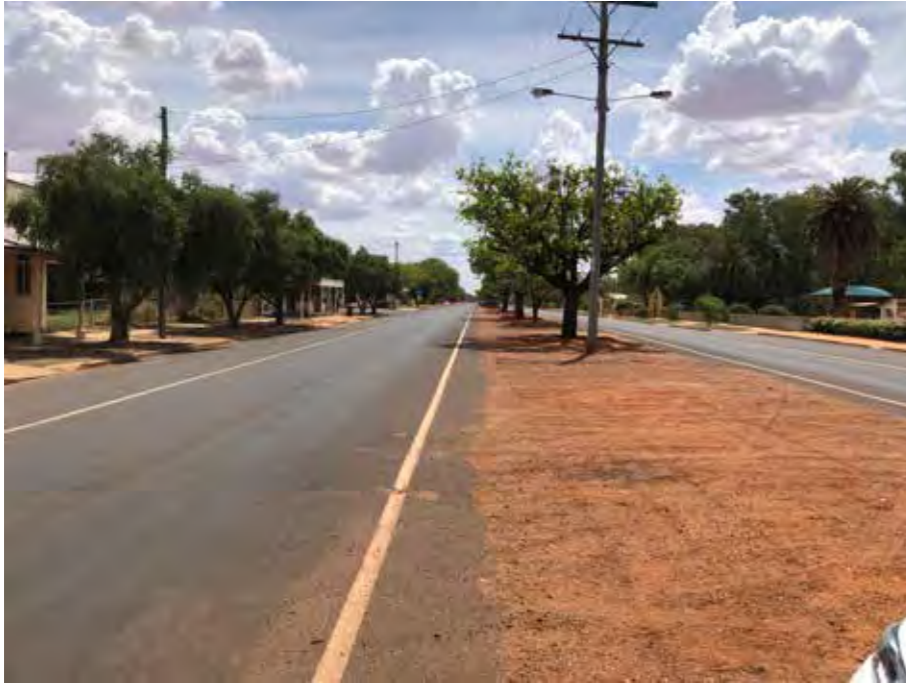
MAIN STREET / BALONNE HIGHWAY
