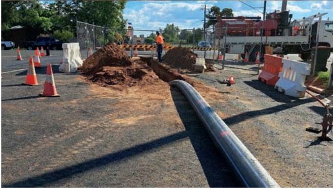
ALFRED STREET WATER MAINS UPGRADE
