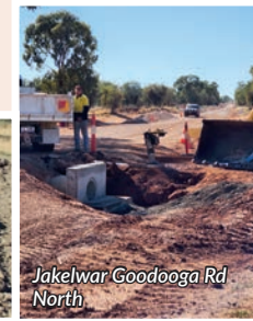
Mungindi Levee Works
