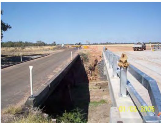
Narran River Bridge
