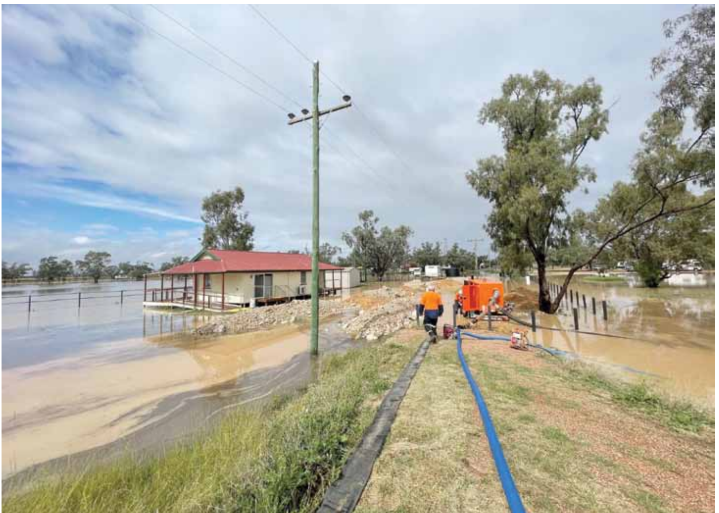
A Council crew at work pumping out water at Thallon.
