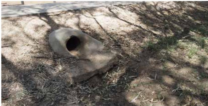
Figure 031. - Insufficient stormwater piping beneath raised pathways causing flow issues and adding to existing erosion issues (Image by Rounsefell Design).
