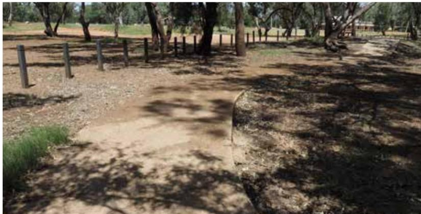
Figure 025. - Low lying existing footpath covered in silt from recent overland flow of rainfall and/or flooding (Image by Rounsefell Design).
